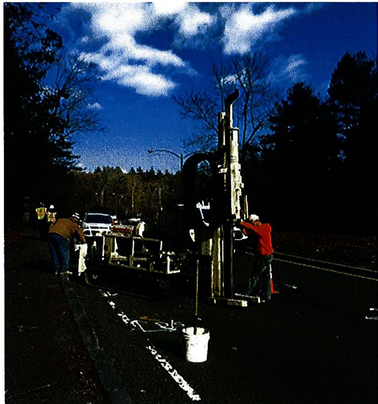
Soil Boring along DCR- Woodland Road
