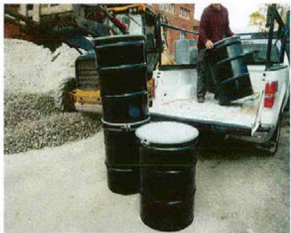
Lead Paint Removal
