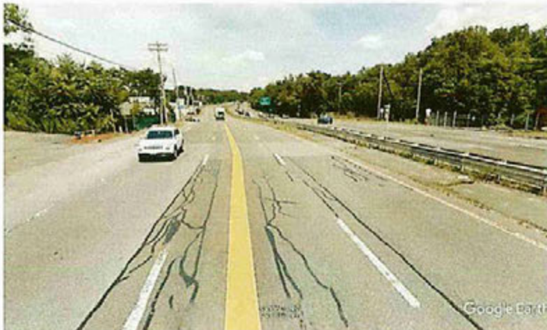
Proposed Pipeline Route in shoulder of Rte. 1 (Looking North)
