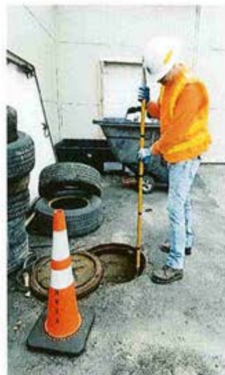
TRAC staff inspect an oil/water separator at an auto repair facility.
