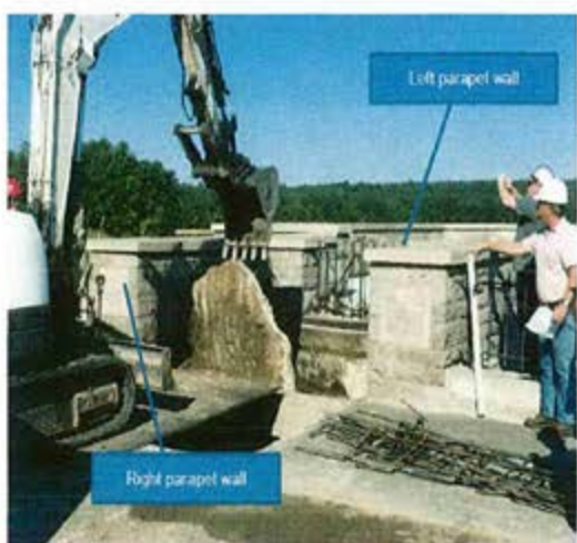
CVA Intake Structure
