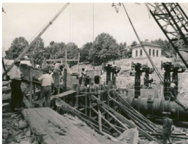
Provisions were left for a future Hultman Connection at Shaft 4
