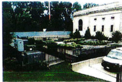
Figure 4: The top of the Emergency Pump Station with the low service condominiums in the background
