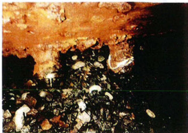
Cap Welded Over Plug
