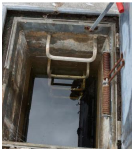
Shaft 7D chamber
