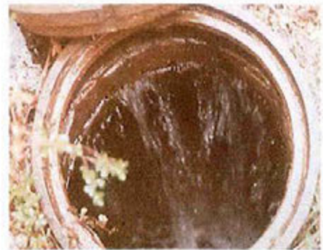
Inflow into a Manhole
