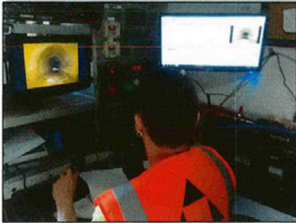
Sewer TV Inspection
