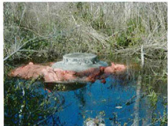
Sewer Manhole in Wetland - Raised and Sealed
