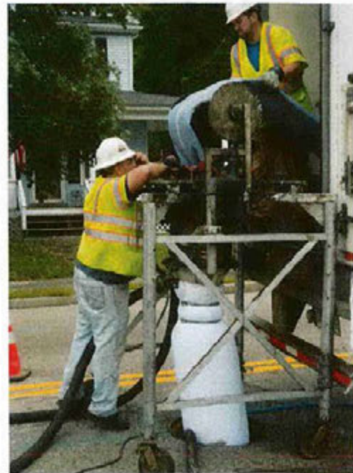
Installation of Cured-In-Place Pipe Liner
