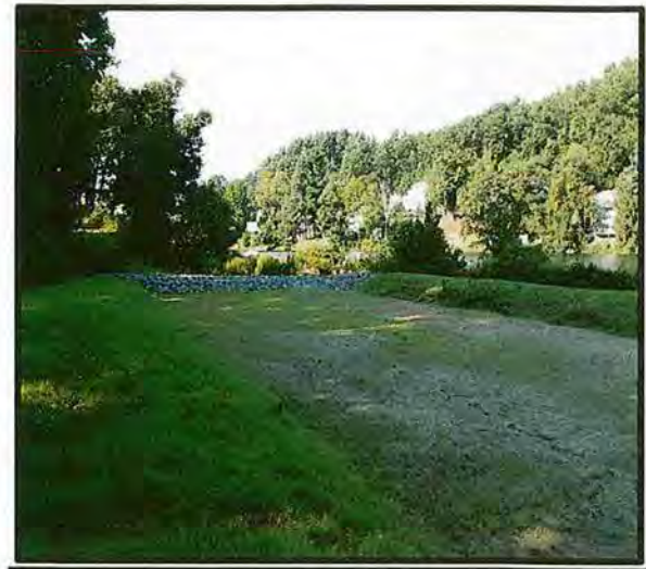
BMP: Grassed bioretention pond for runoff collection and treatment under Phase I
