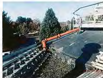
View of fixed cover digester roof from Digester Building roof
