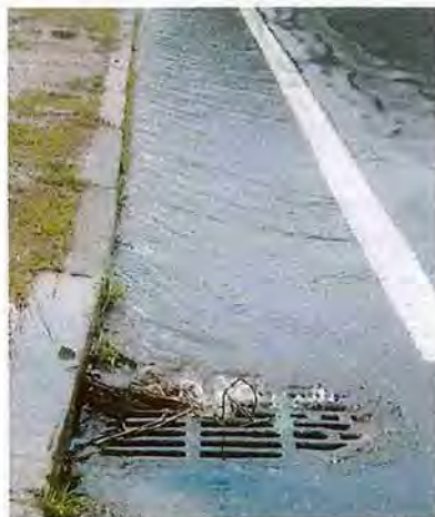
Highway catch basin
