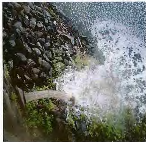
Catch basin discharge point in reservoir
