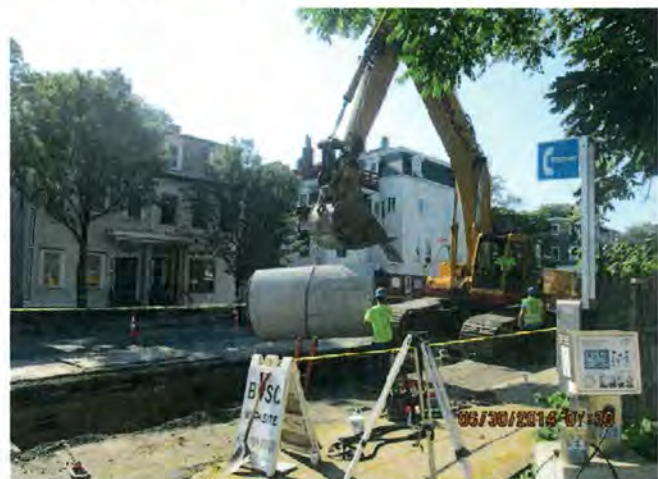
48-inch drain installation on L Street, Contract 4
