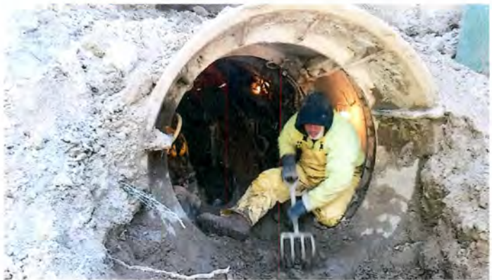
Pipe jacking under Woodland Road
