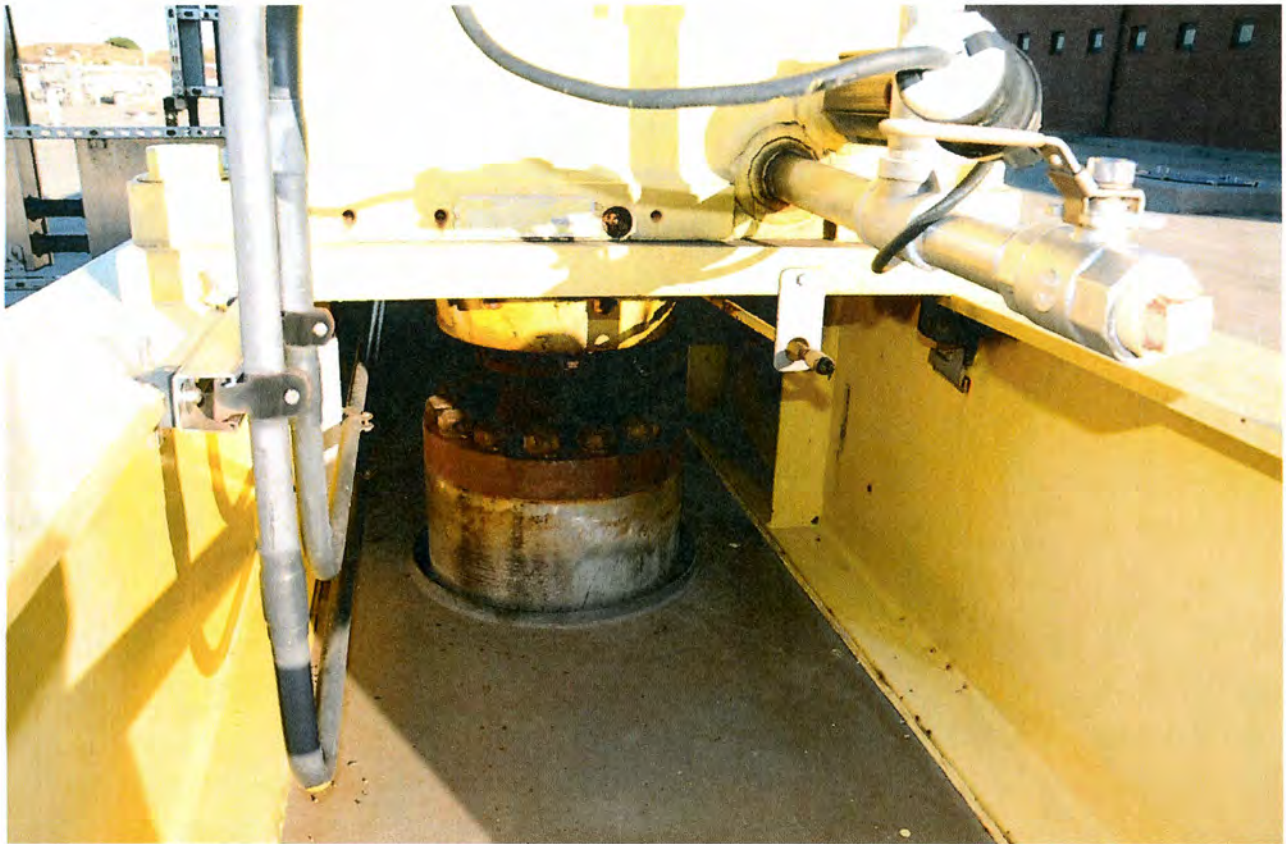
Picture depicts the top of one of the aerator/mixer shafts where it connects with the triple-reduction gearbox
