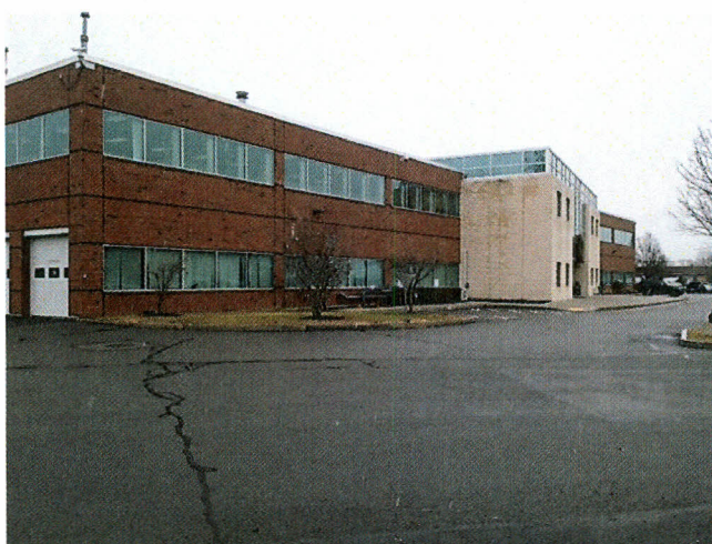
Chelsea Administration Building
