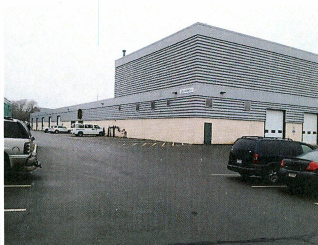
Chelsea Maintenance Building
