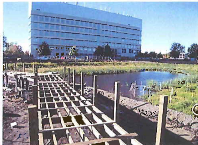
Figure 4: Framing of boardwalk across main basin
