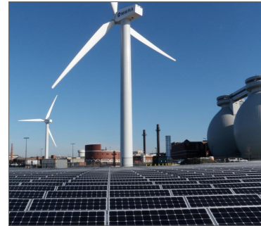
Wind turbines and solar panels at the Deer Island Wastewater Treatment Plant
