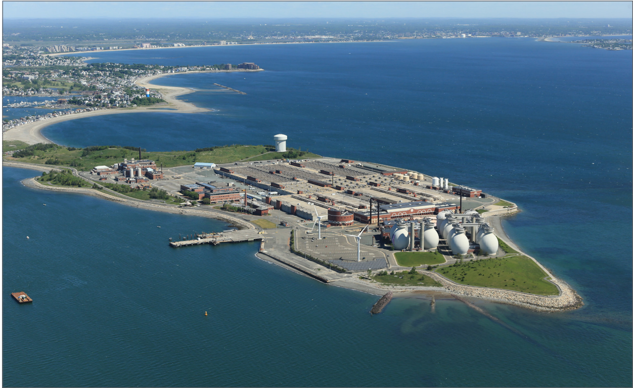
Deer Island Wastewater Treatment Plant
