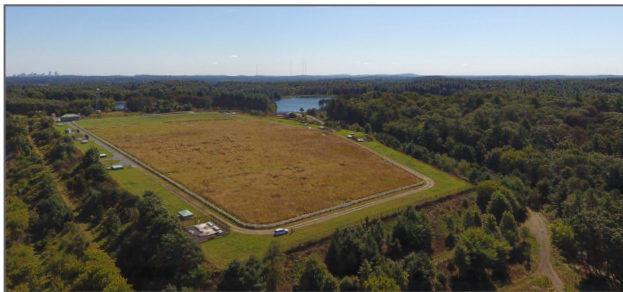
Norumbega Covered Storage Facility in Weston
