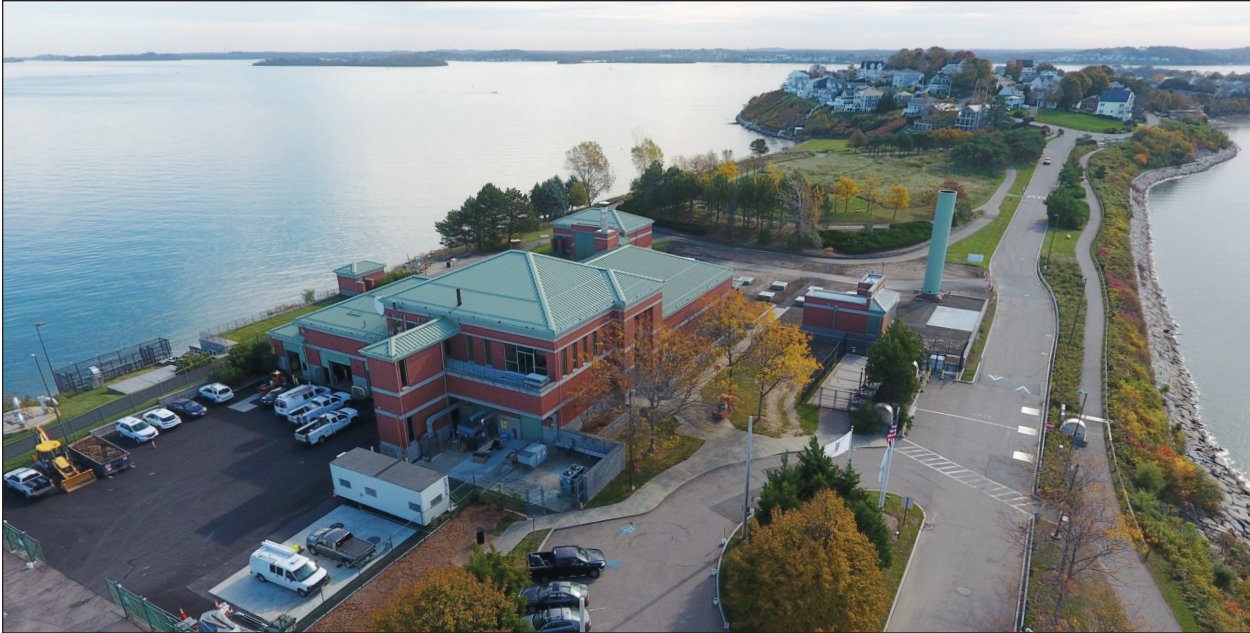
Nut Island Headworks
