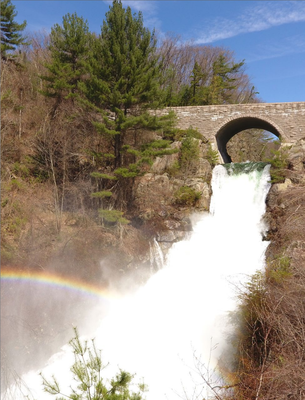
Quabbin Reservoir Spillway
