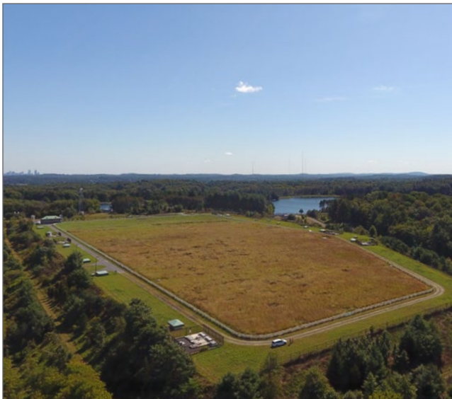
Norumbega Covered Storage
