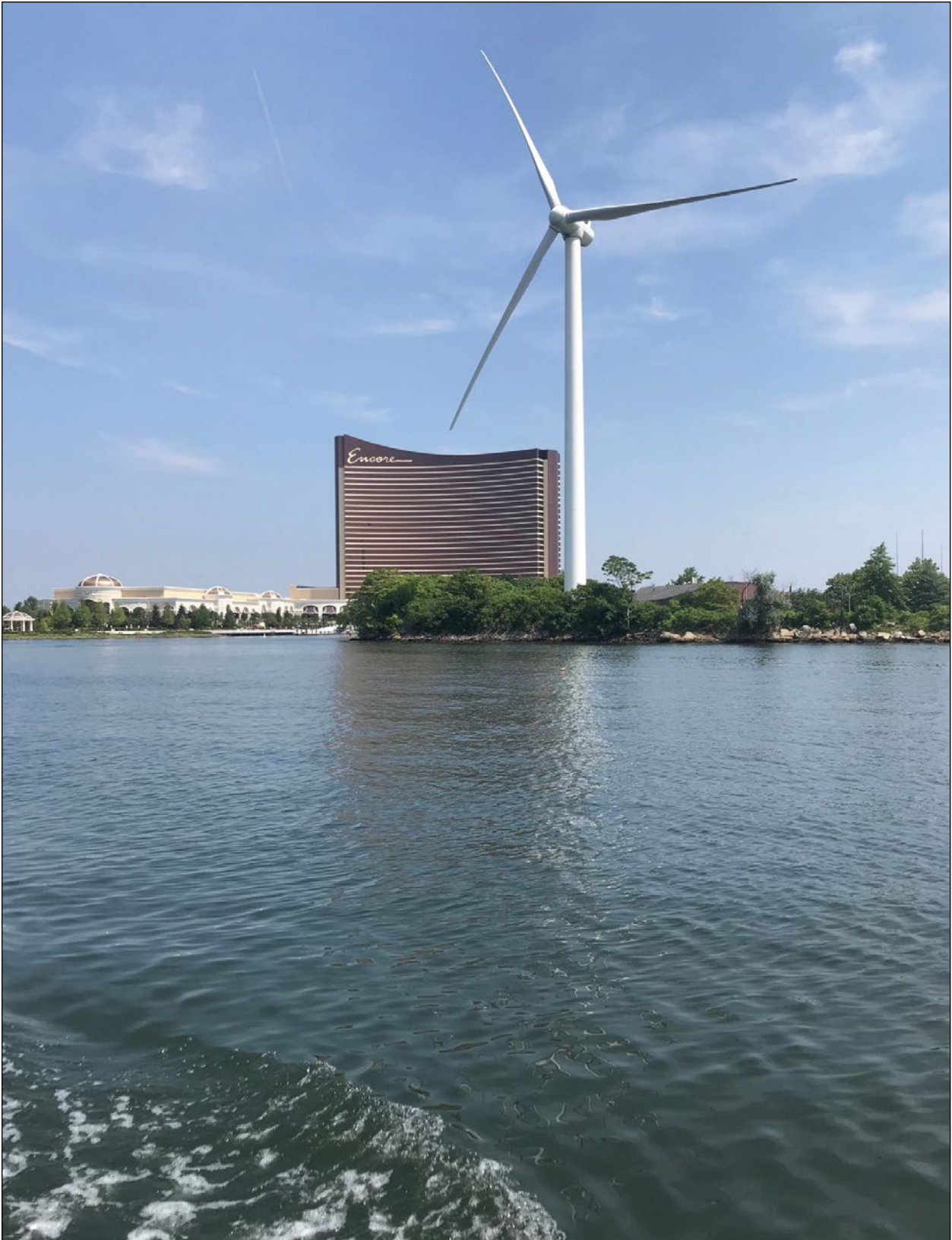
Charlestown Wind Turbine
