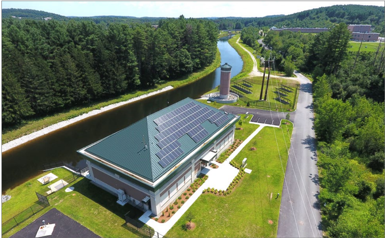
Wachusett Aqueduct Pumping Station
