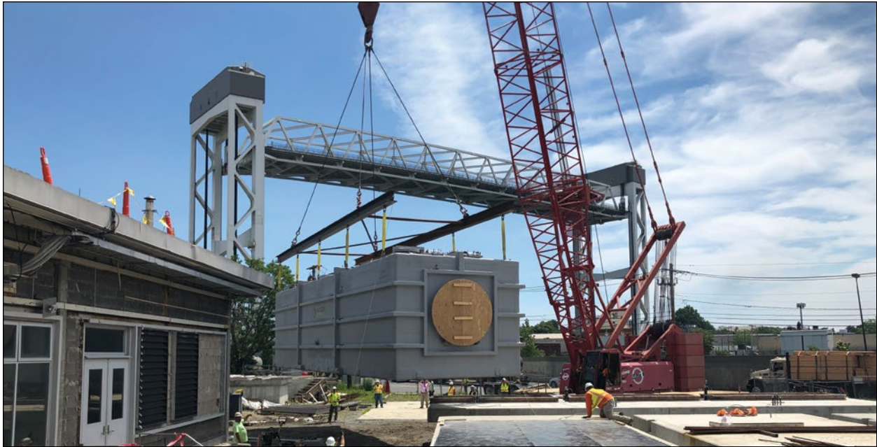
Chelsea Creek Headworks
