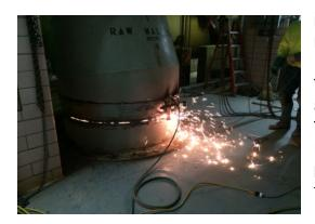
North Main Pump Station and Winthrop Terminal Facility Butterfly Valve Replacement - \$3.5 million FY18 spending (\$17.5 million total construction cost). This project will replace butterfly valves in the NMPS and eight 36-inch plug valves in the Winthrop Terminal Facility, for isolating the pumps when maintenance is required. Also includes replacement of primary sludge piping and eight hydraulic actuators for the South System Pump Station check valves.
