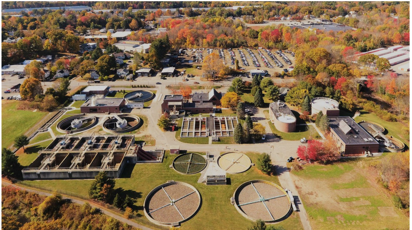
Clinton Wastewater Treatment Plant
