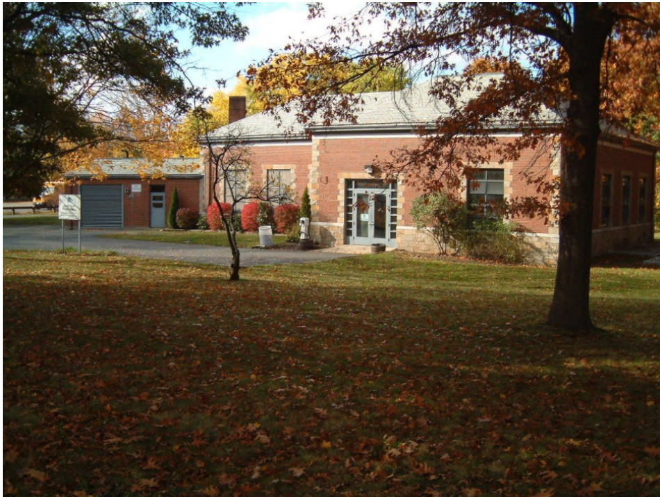
Alewife Brook Wastewater Pump Station
