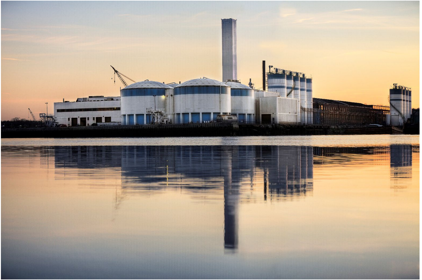
MWRA Sludge Pelletizing Facility
