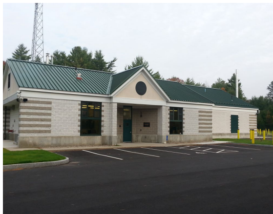
Brutsch Water Treatment Facility
