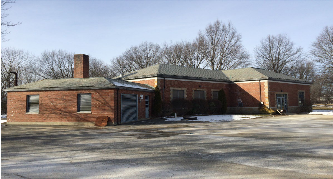
Alewife Brook Wastewater Pump Station
