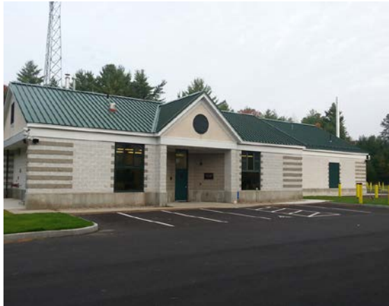
Brutsch Water Treatment Facility
