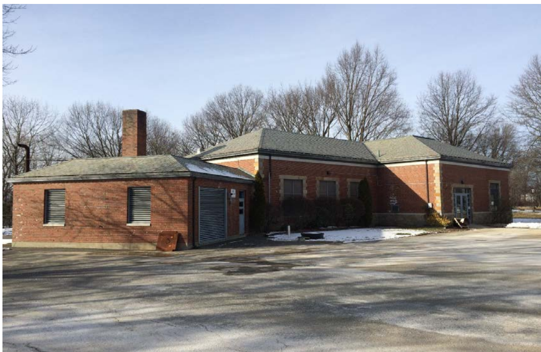
Alewife Brook Wastewater Pump Station
