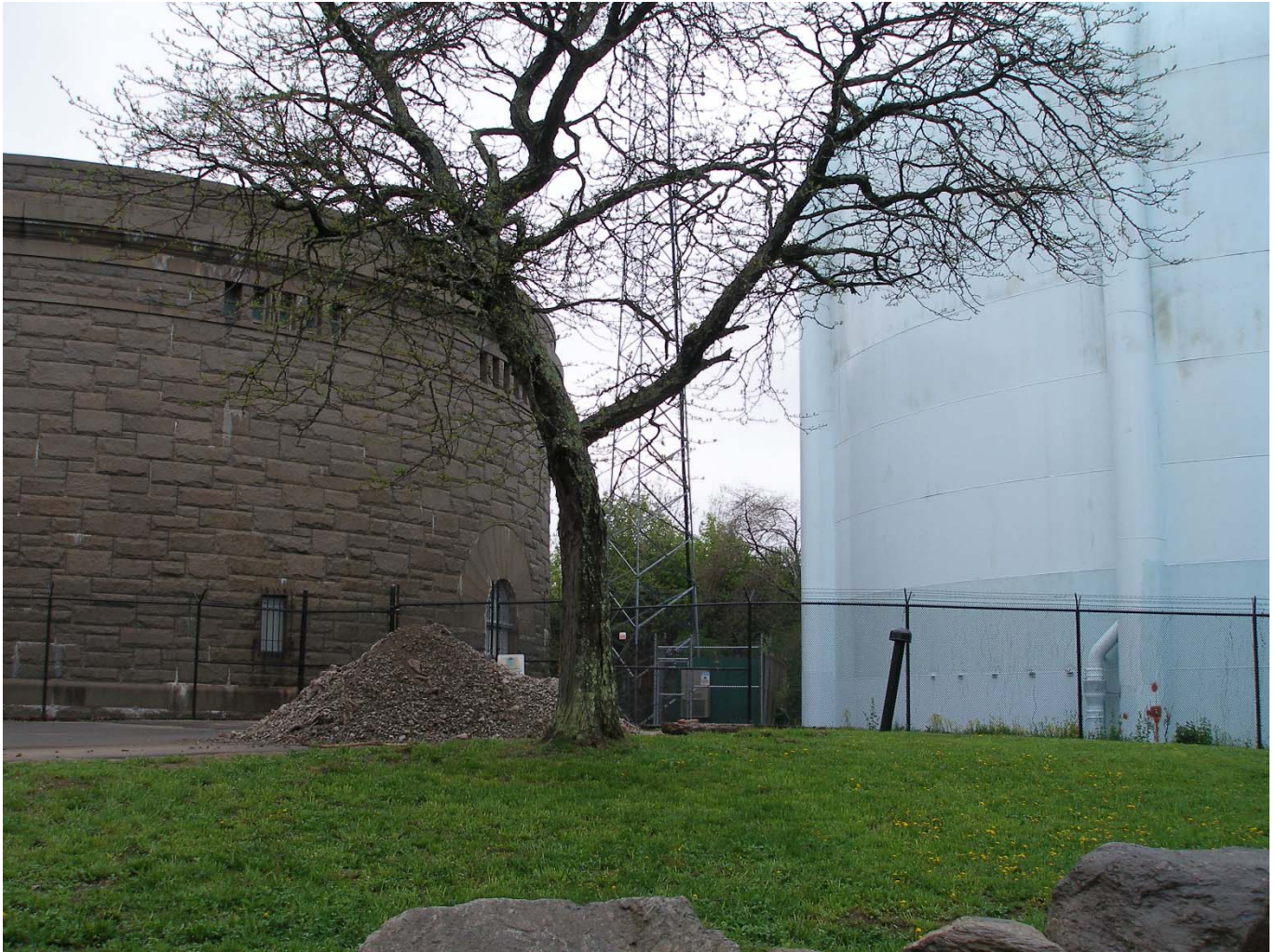
Bellevue Storage Tanks
