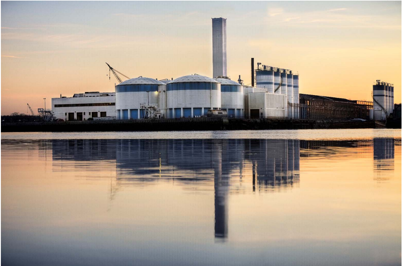
MWRA Sludge Pelletizing Facility
