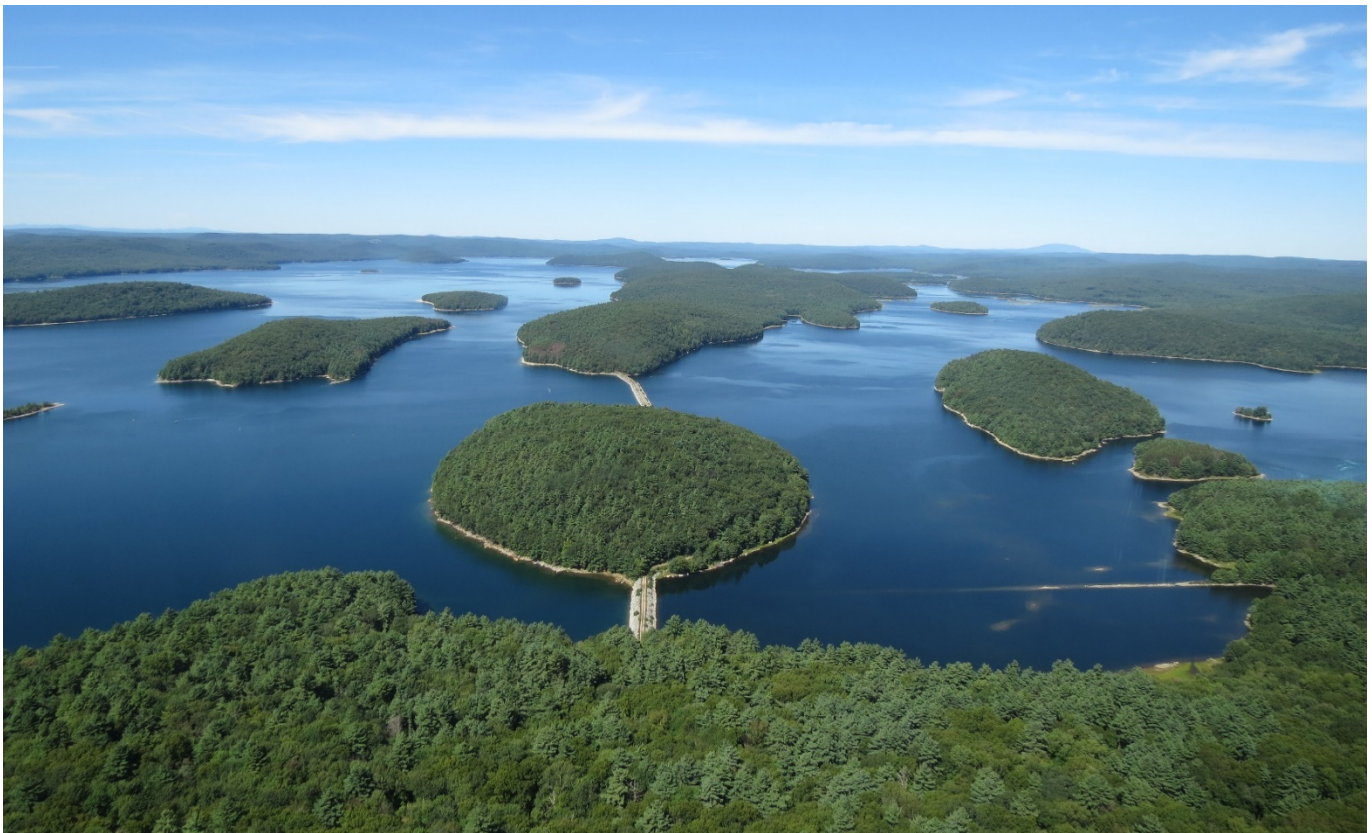
Baffle Dams Quabbin Reservoir
