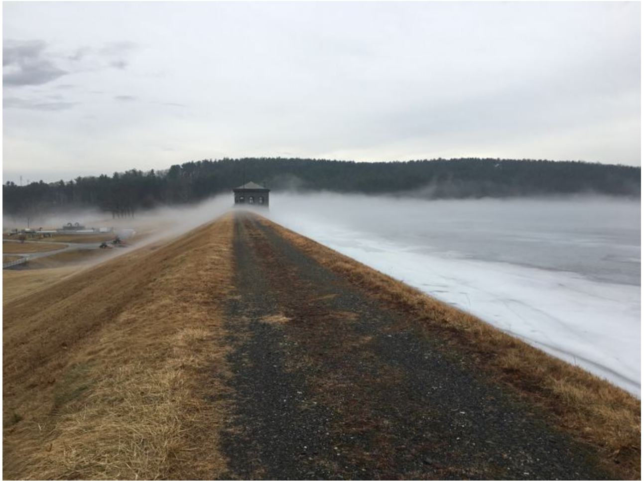
Fog creeping in over Sudbury Dam
