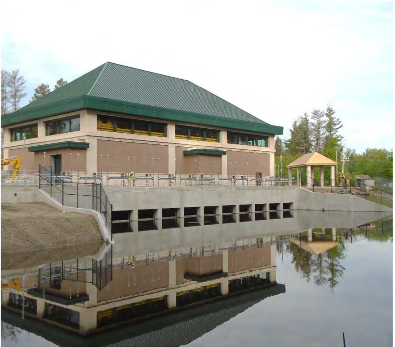
Wachusett Aqueduct Water Pump Station Forebay
