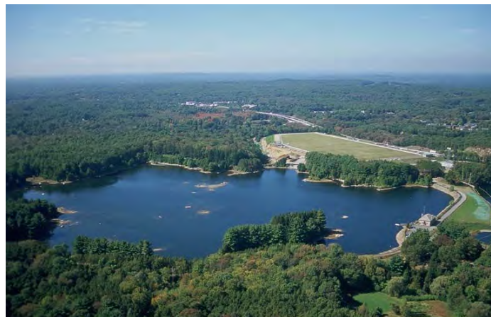
Norumbega Covered Storage Tank
