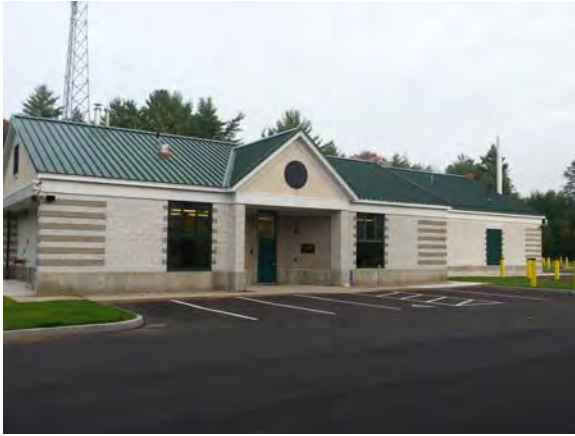
Brutsch Water Treatment Facility
