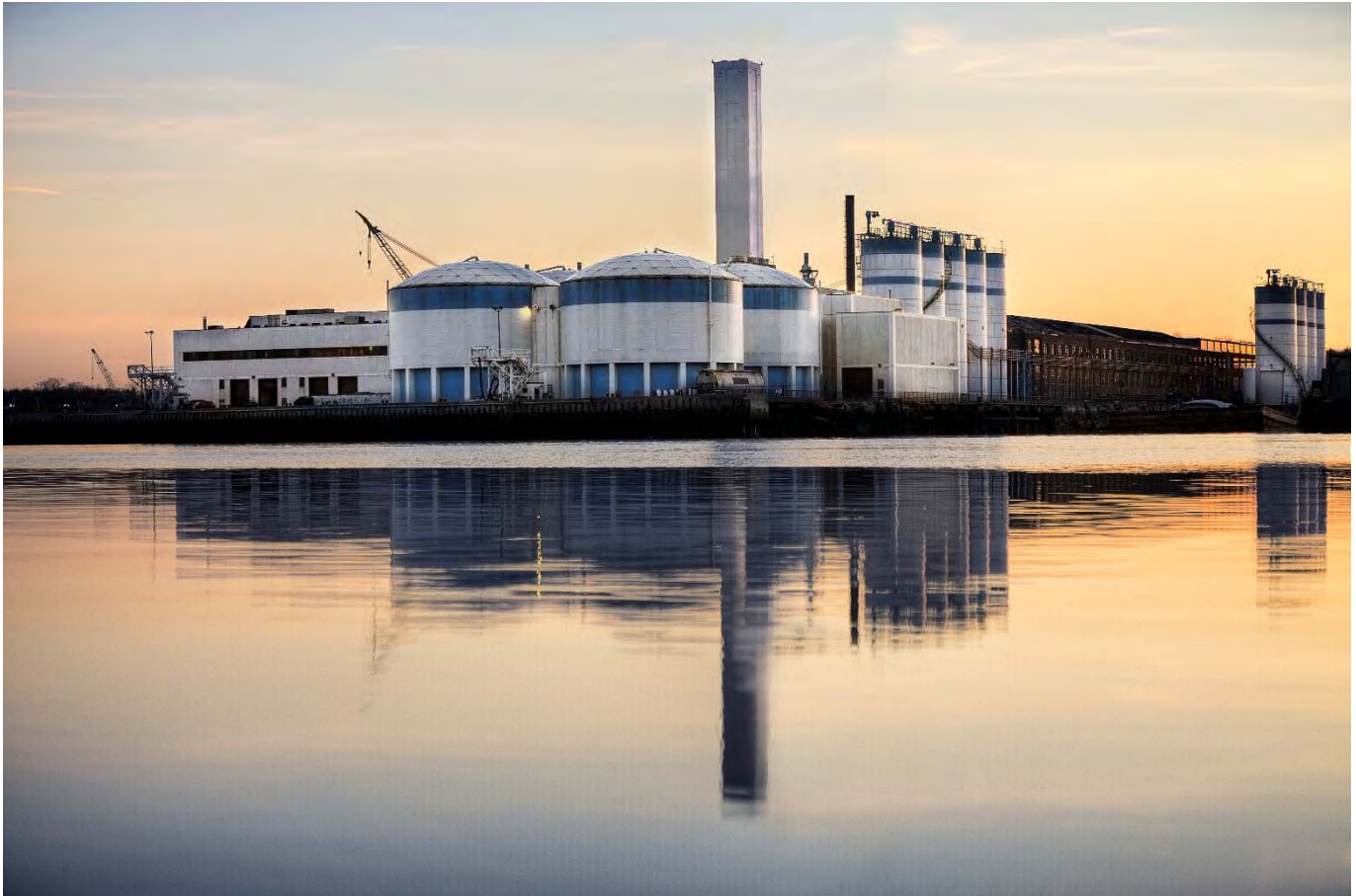
MWRA Sludge Pelletizing Facility
