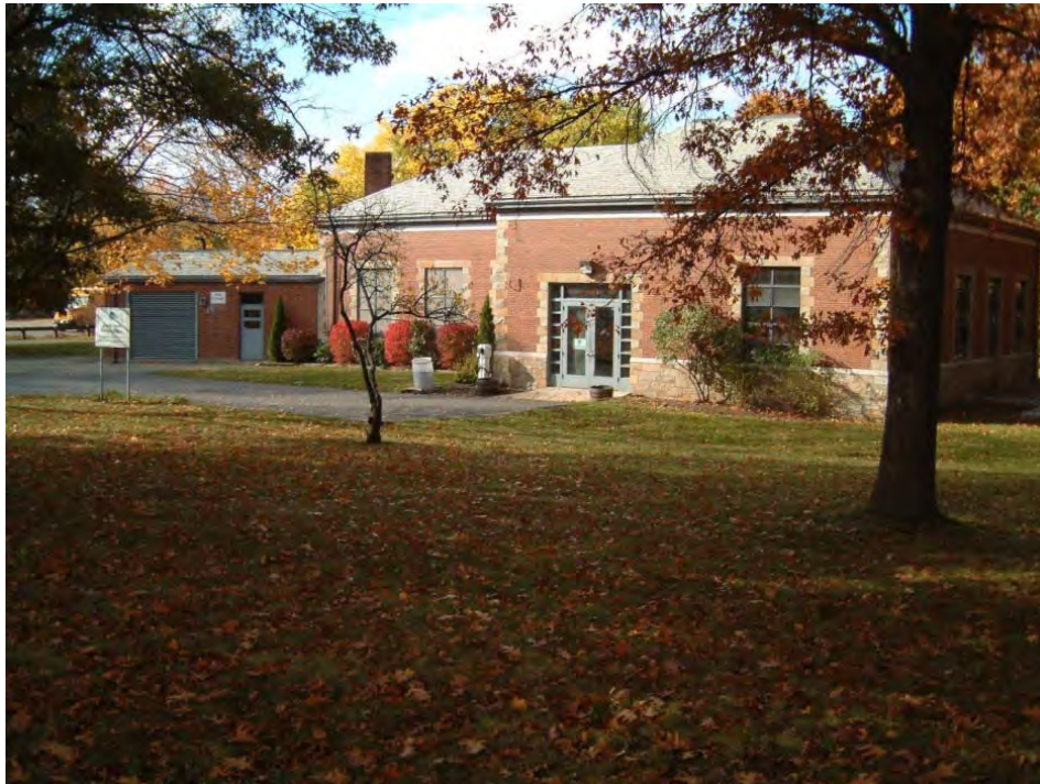
Alewife Brook Wastewater Pump Station
