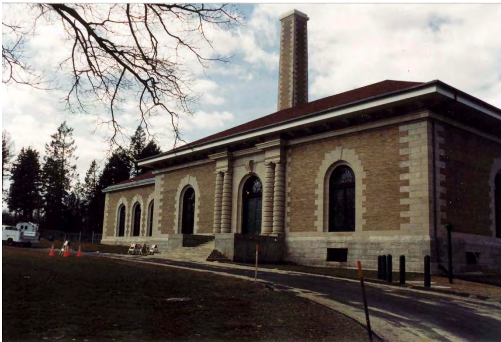
Gillis Water Pump Station
