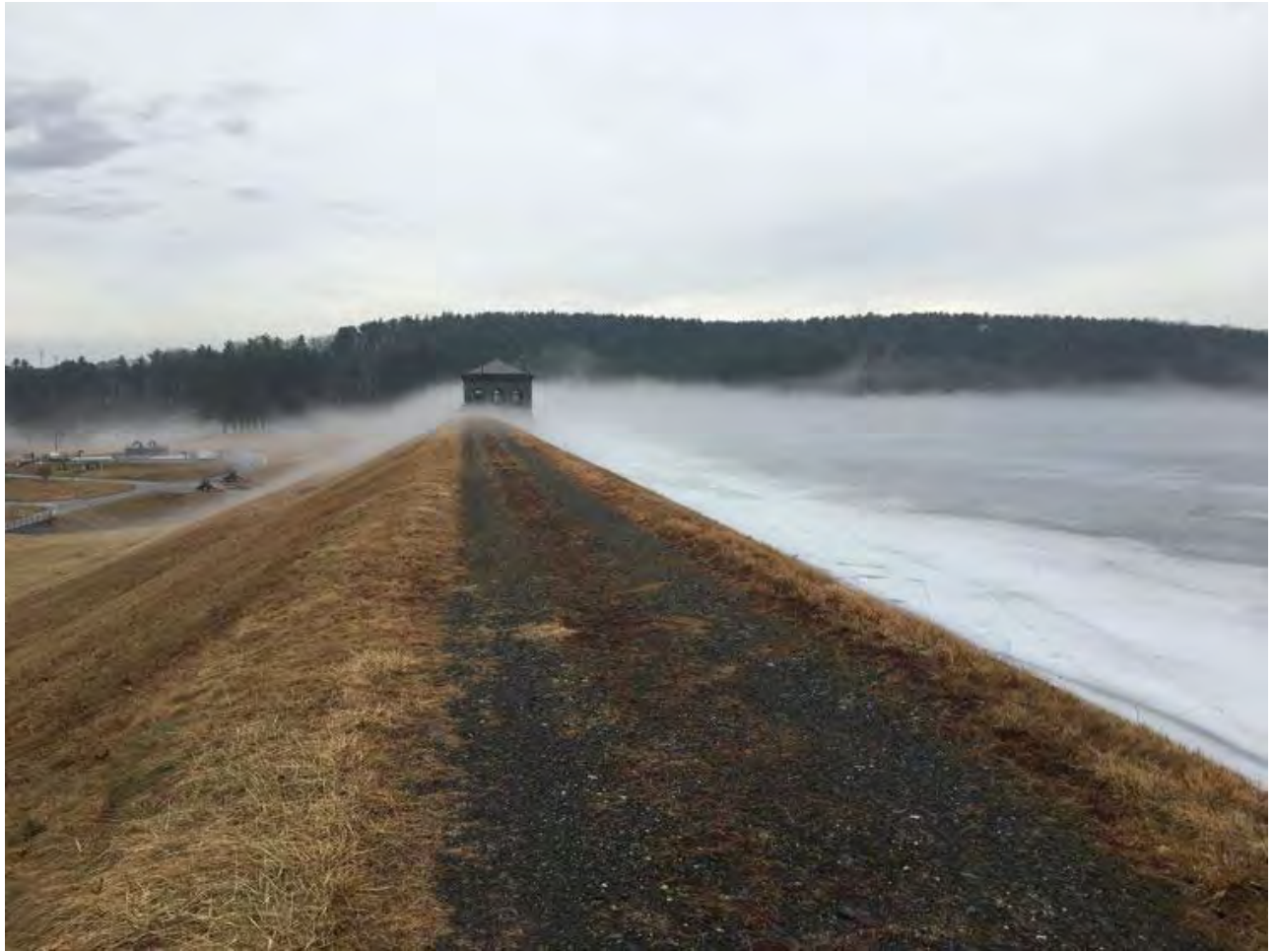
Fog creeping in over Sudbury Dam
