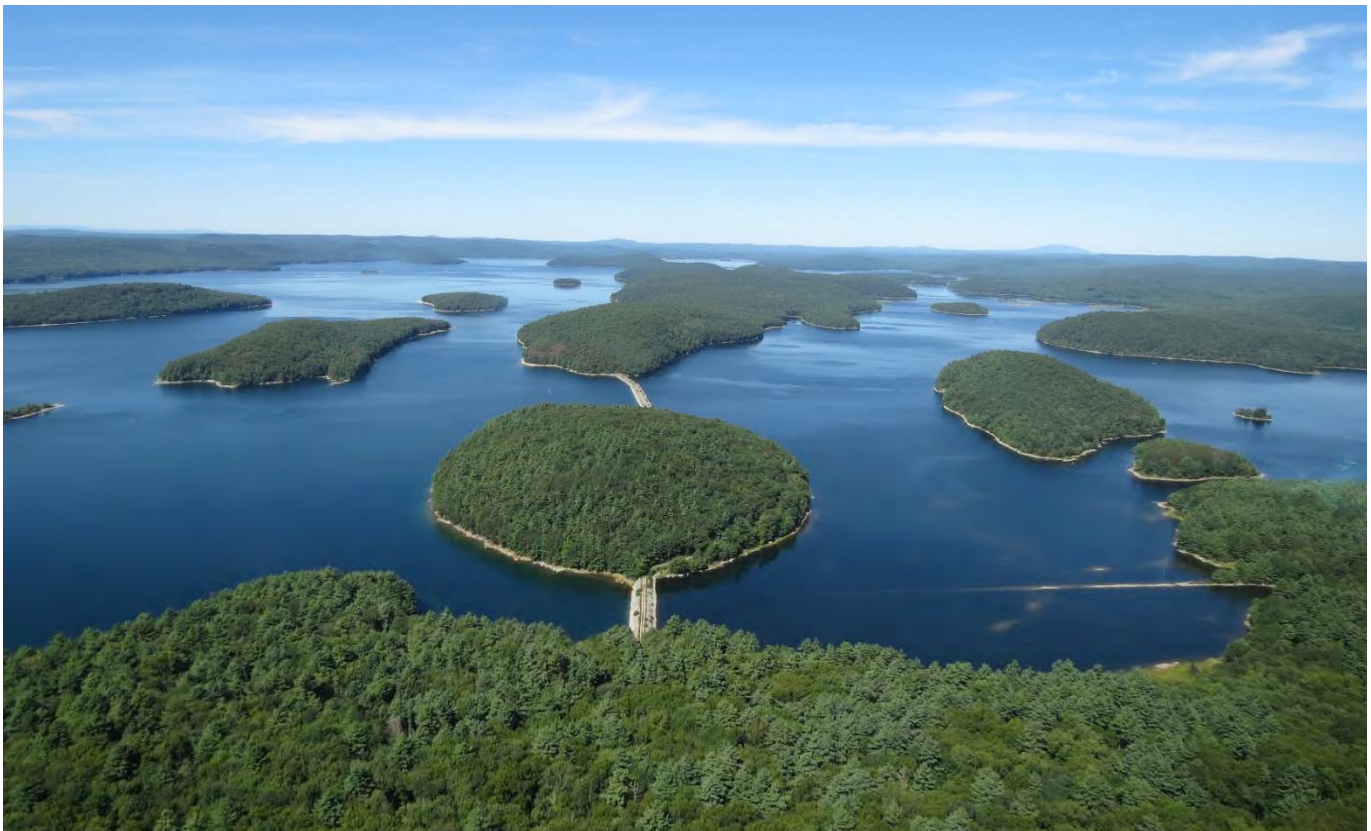
Baffle Dams Quabbin Reservoir
