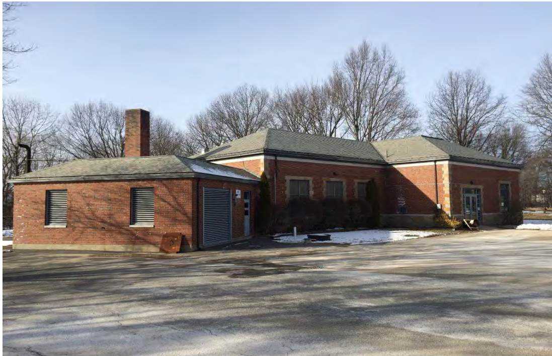
Alewife Brook Wastewater Pump Station
