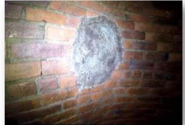
SOM002 Weir Closed
