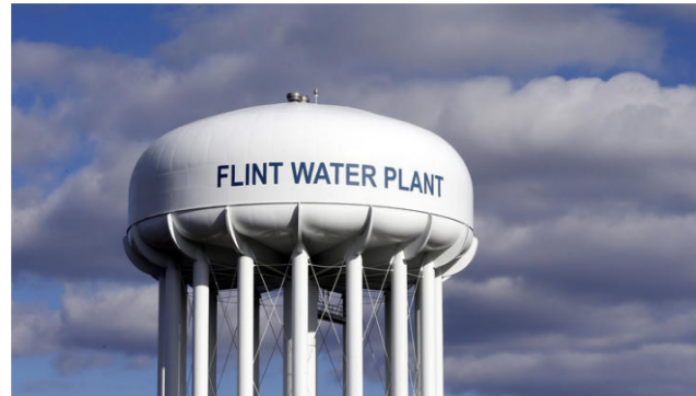
Flint will replace at least 18,000 lead or galvanized-steel water lines by 2020, and the state will pick up the bill with state and federal money. (Carlos Osorio / AP)
