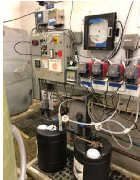
Figure 1: Inspecting Pretreatment System
