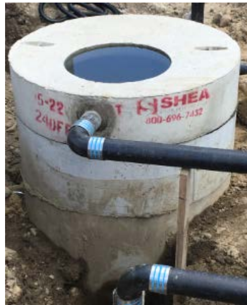
Figure 2: New trap inspection
