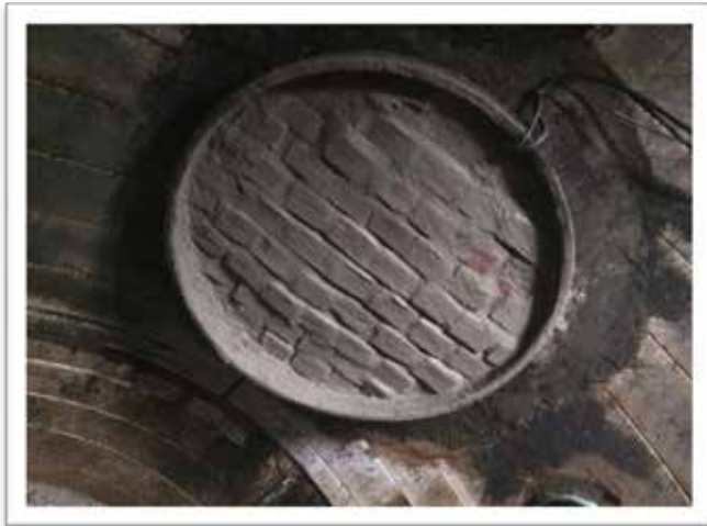
Brick and mortar bulkhead of high outlet overflow in CSO regulator at Outfall CHE002.
