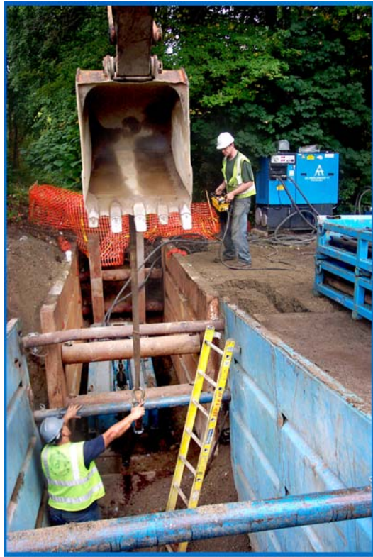
Typical set up for pipebursting operation.
