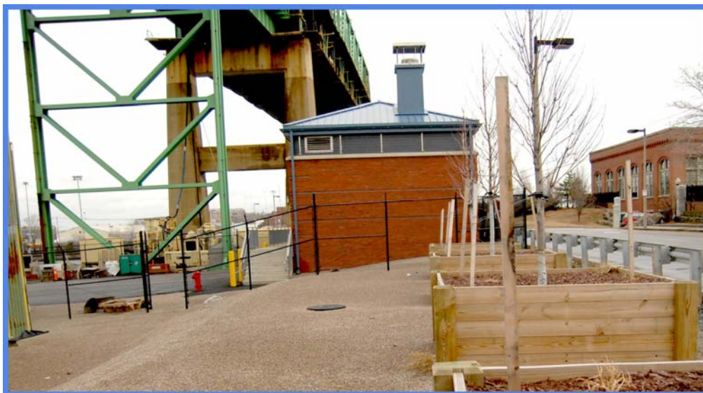
Completed Pump-Out/Odor Control Facility Above CSO Storage Tunnel
