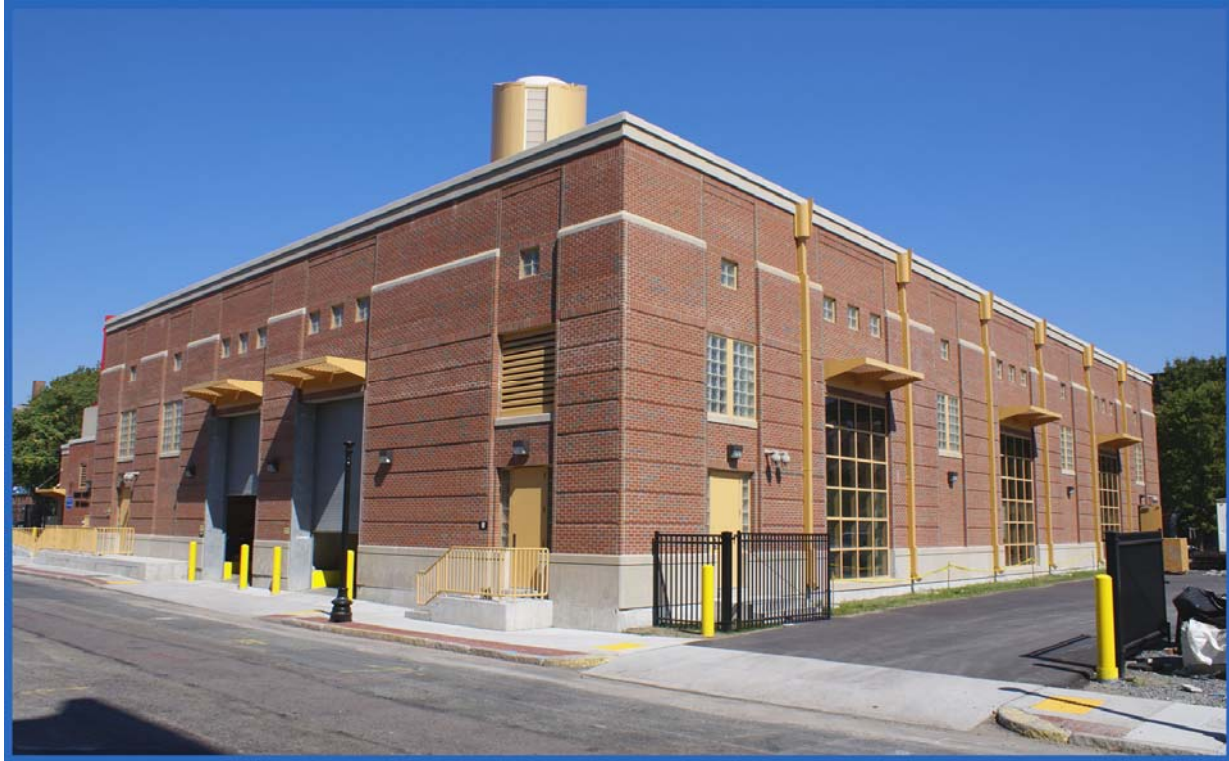
Union Park Detention and Treatment Facility, South End, Boston
