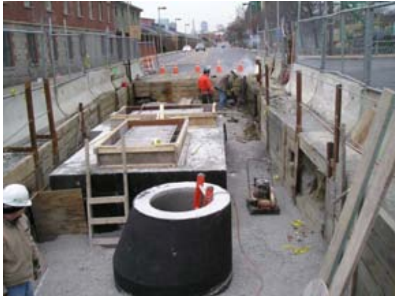
Construction of BOS019 CSO diversion structure in Chelsea Street
