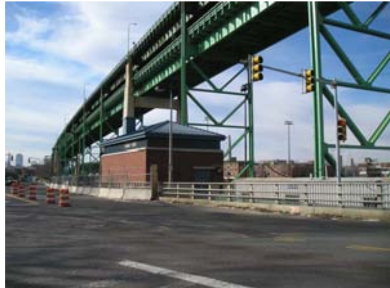
New pump station to dewater the BOS019 storage conduit
