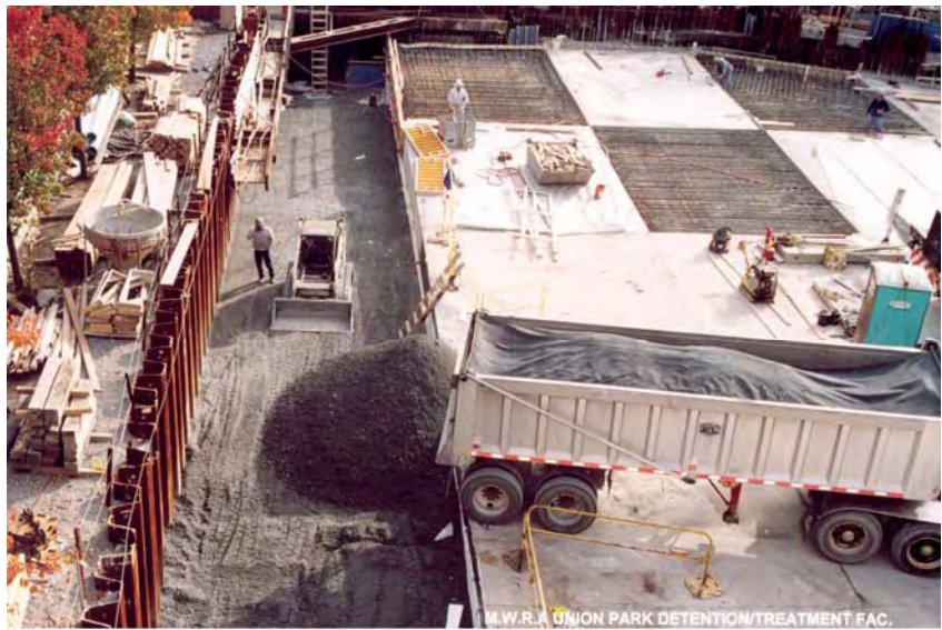
Backfilling operations on the roof slab over the effluent channel
