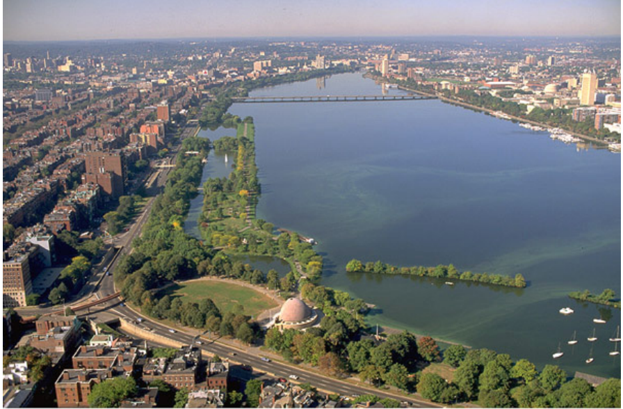
On the Charles River, MWRA has eliminated or greatly reduced CSO discharges at several outfalls along the Esplanade and has upgraded the Cottage Farm CSO Treatment Facility to improve disinfection and provide dechlorination, while BWSC continues construction of a sewer separation project that will minimize CSO discharges to Stony Brook.
