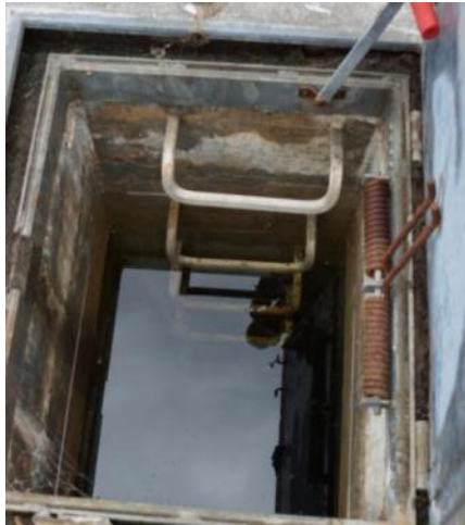
Shaft 7D chamber
