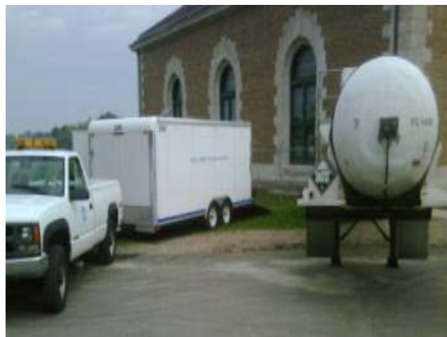
Mobile disinfection unit and chlorine tank at Gillis Station
