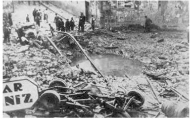
WW II Bomb crater in England, water leaking from broken main
