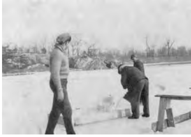
1966 Copper sulfate dosing through ice using a hole and an outboard motor
