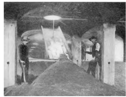
1918 Providence RI slow sand filter interior
