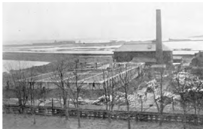
1910 Newport RI Water Treatment Plant
