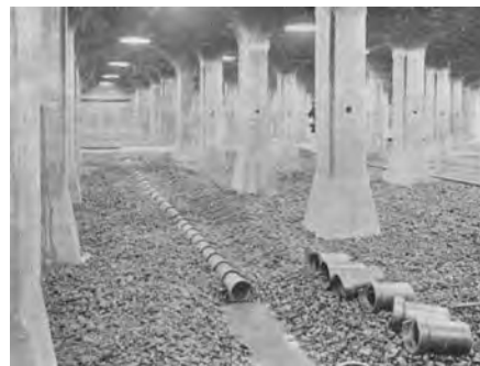
1918 Providence RI slow sand filter interior
