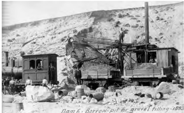
1893 Excavation for Sudbury Reservoir Dam
