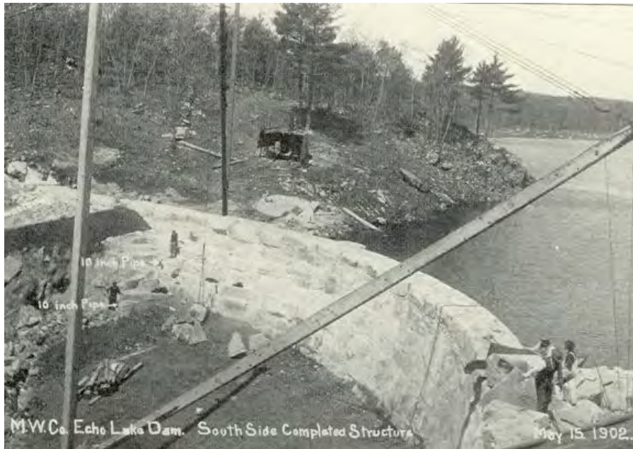
1902 Milford MA Masonry Dam
