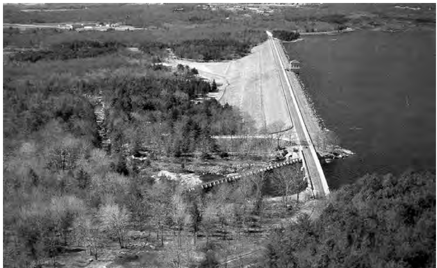
1922 Gainer Dam at Scituate Reservoir, Providence RI supply
