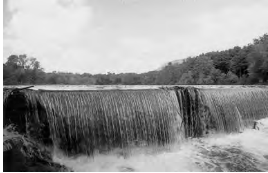
1860 Lake Whitney Dam serving New Haven CT
