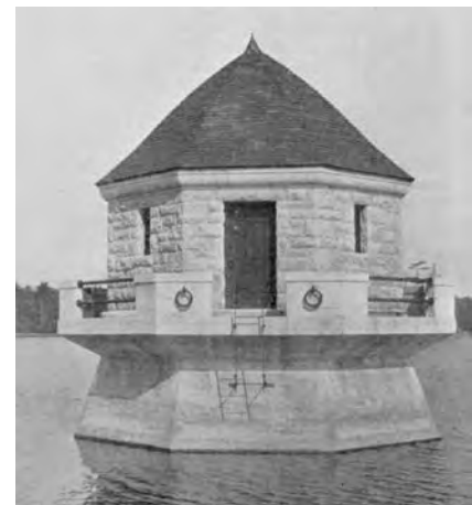
1925 New Bedford deep intake on Quitticas Pond
