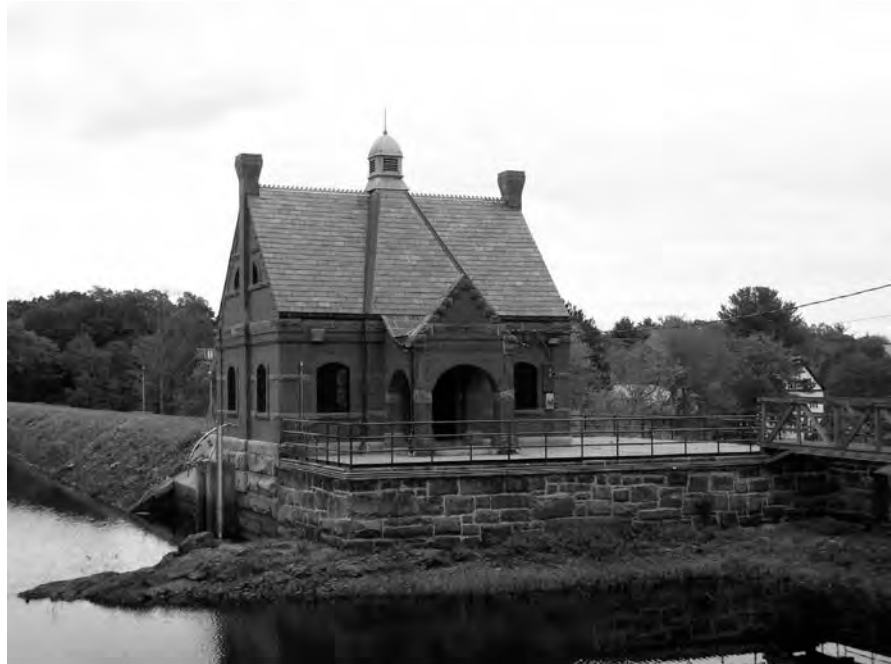
1887 Cambridge's Stony Brook Dam and Gatehouse, Waltham MA
