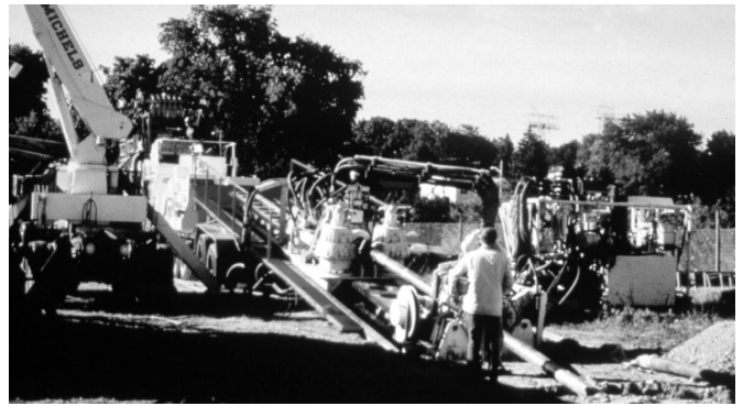
The Horizontal Directional Drilling procedure, shown here at Mill Cove in 1997, begins with the horizontal drilling of an 8-inch diameter pilot hole. The hole is then enlarged until it reaches its ultimate diameter. Finally, the pipeline is pulled through the reamed hole.
