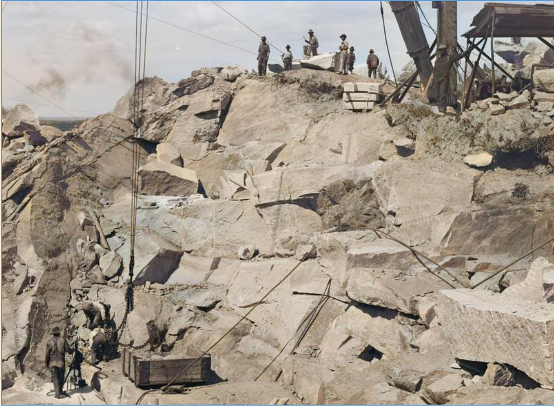
Getting out rock at the Quarry involved the lifting, over the heads of other workers, of heavy loads with a derrick (crane).
