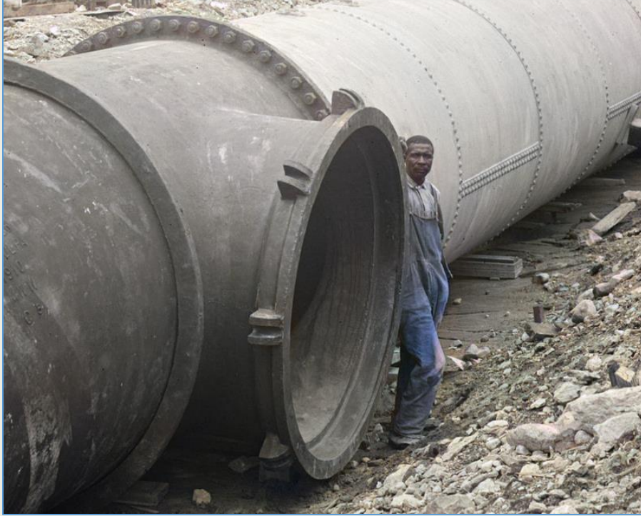
A pipe layer on a short break.
