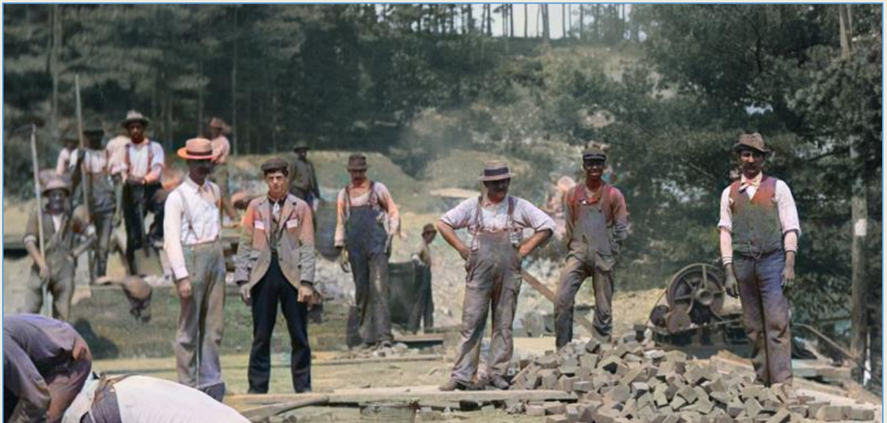
A crew laying brick arches at the Assabet River Bridge.
