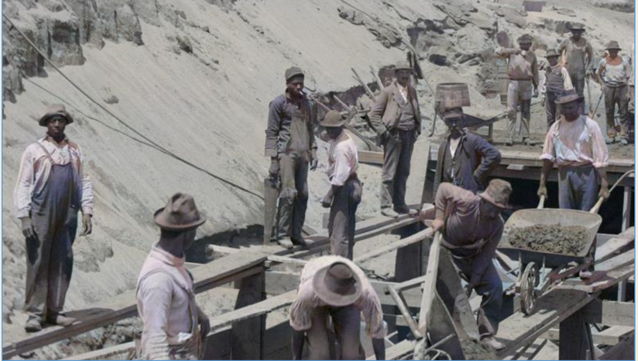
A work gang forming and pouring concrete.
