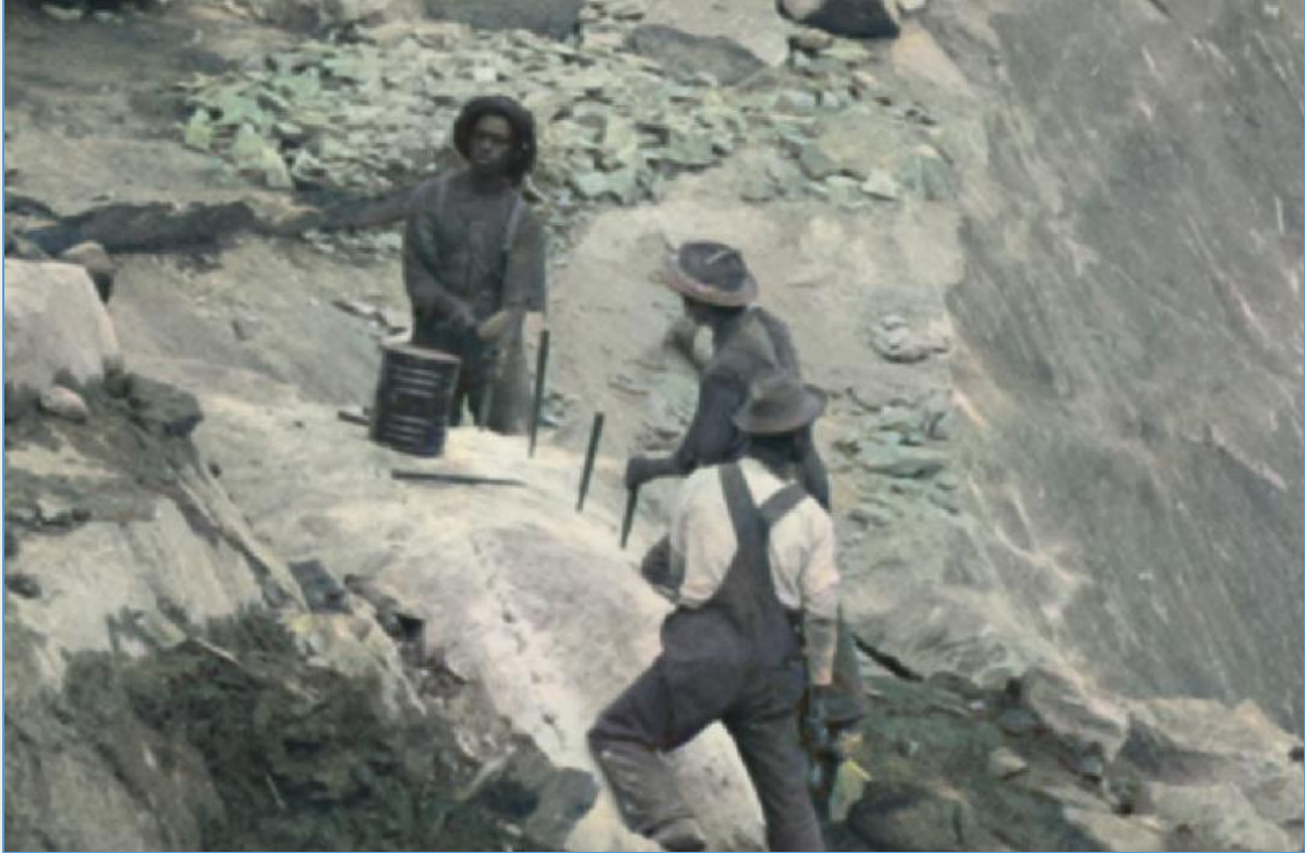
After the blast, huge rocks are split by hand into manageable pieces with old fashioned wedges.
