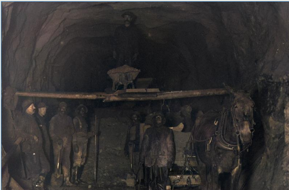
Tunnel excavation crew.
